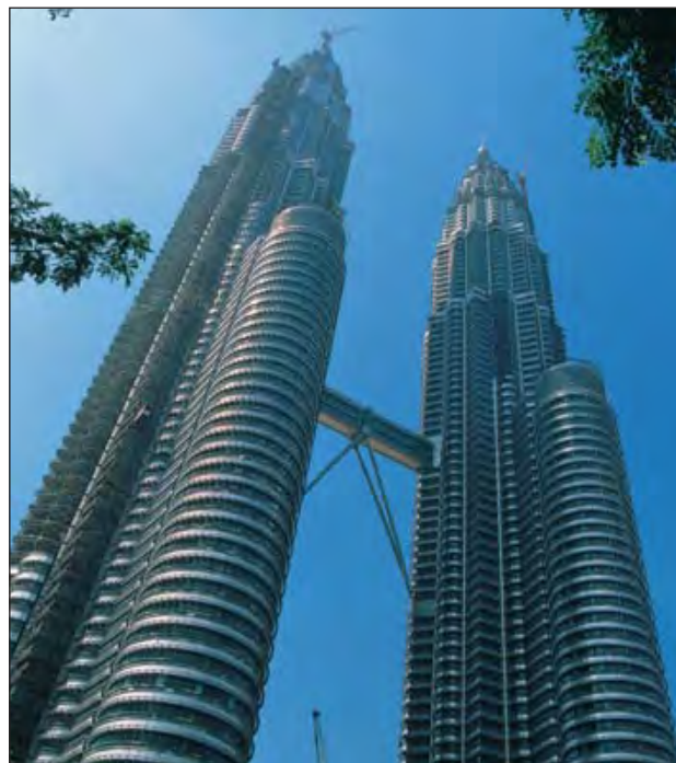
Furse has extensive experience of designing and supplying lightning protection systems for tall structures, including Petronas Towers, Malaysia and many new developments in the Far East
